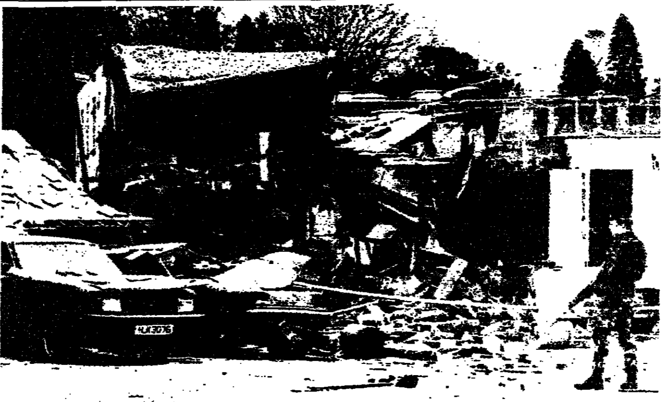
Economic warfare: The Inn on the Park at Dungannon, severely damaged by a car bomb.
